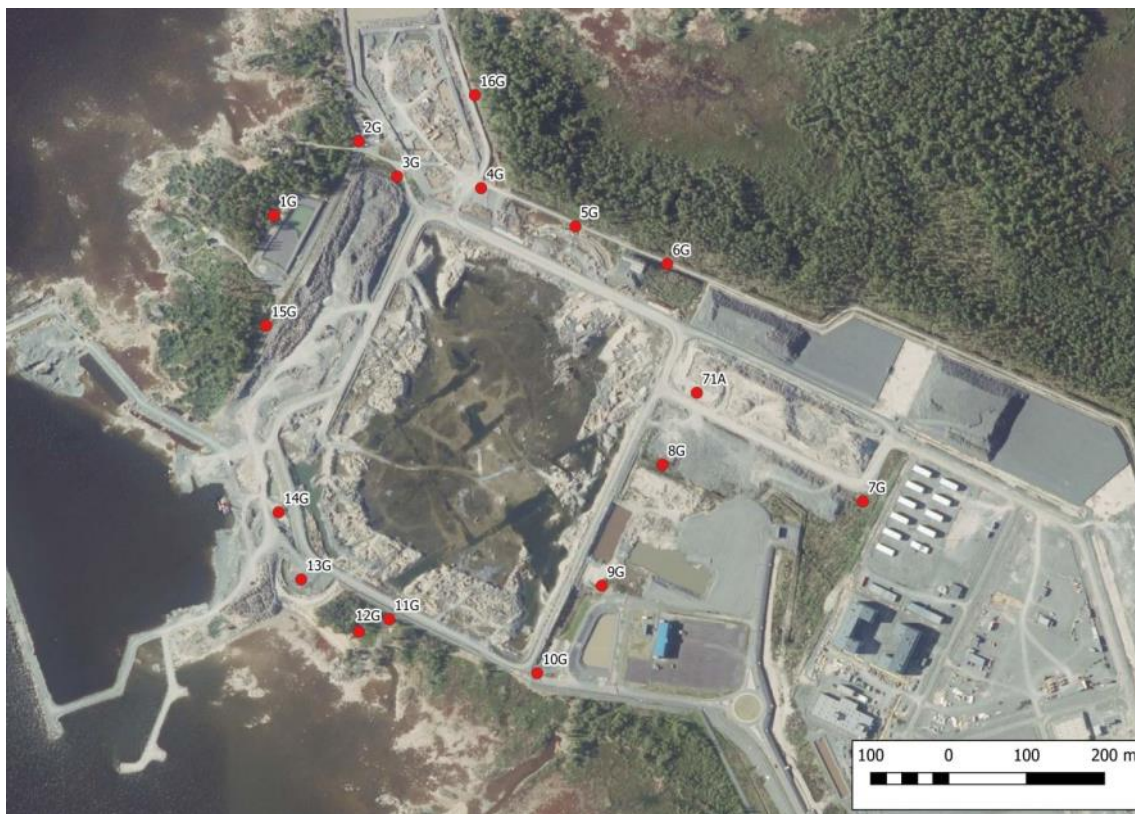
Figure 5. Location of groundwater monitoring wells around construction area (Eurofins Ahma Oy, 2019-2021)
