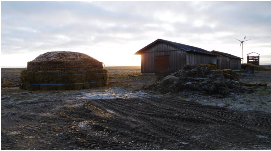
Söderfjärden Meteorita Visiting Center with the new biomeiler (Photo: Novia UAS)
