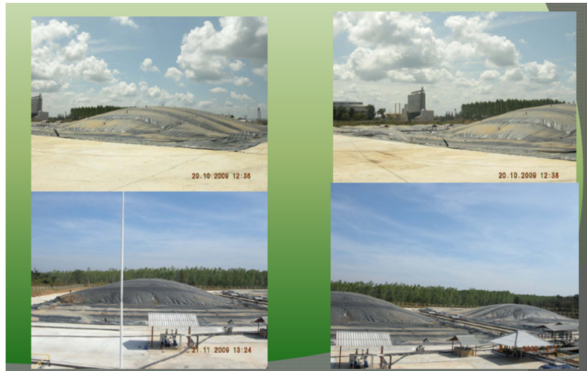
FIGURE 24. Operating covered lagoon building (MoIT, 2013)
