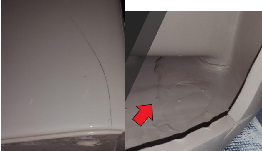
Figure 47: Hairlike crack from pressure feed (Source: Robert Kallström)
