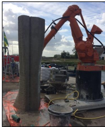
Figure 4. fixed robotic system for 3DCP (CyBe Construction 2022)
