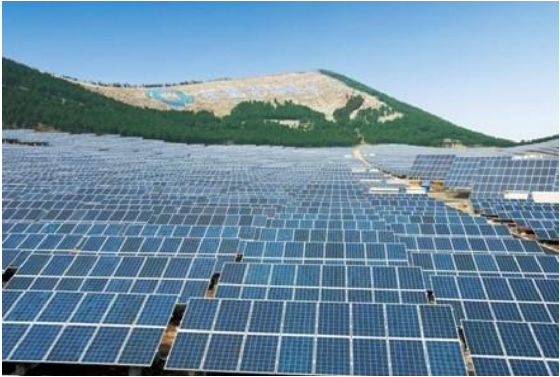
Figure 3.2 Huanghe Hydropower Golmud Solar Park [W5]
