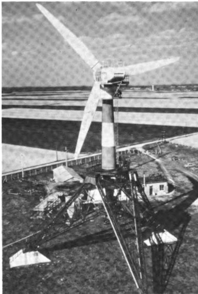
Figure 2. French wind turbine located near Paris, France; 800 kW (36 mph rated wind speed)
