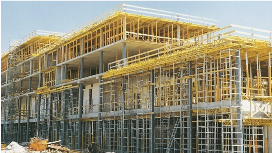
Figure 17. Formwork of a project (Uzodimma, 2020).
