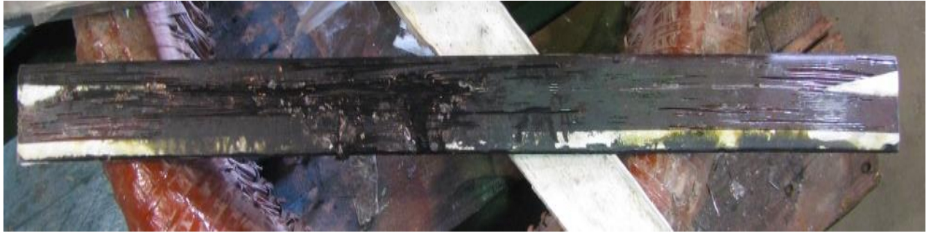
Figure 21. Slot insulation failure.
