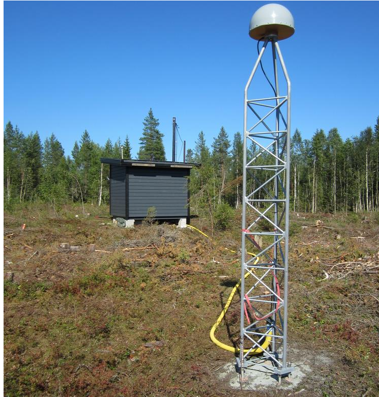
Figure 37. TORN station in summer 2013, showing the antenna mast and the station cottage. (Finnish Geodetic Institute, n.d.)
