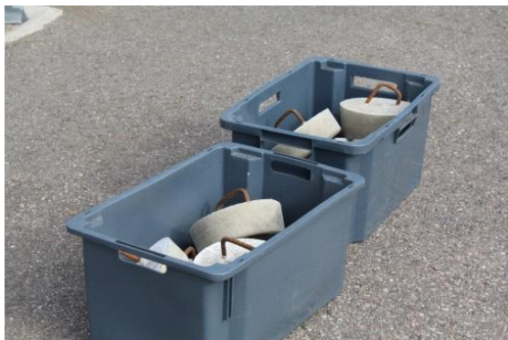
Picture 1. Construction of the mooring buoys is starting. Bottom weights for the guidelines loaded into the box © Hanna Halonen
