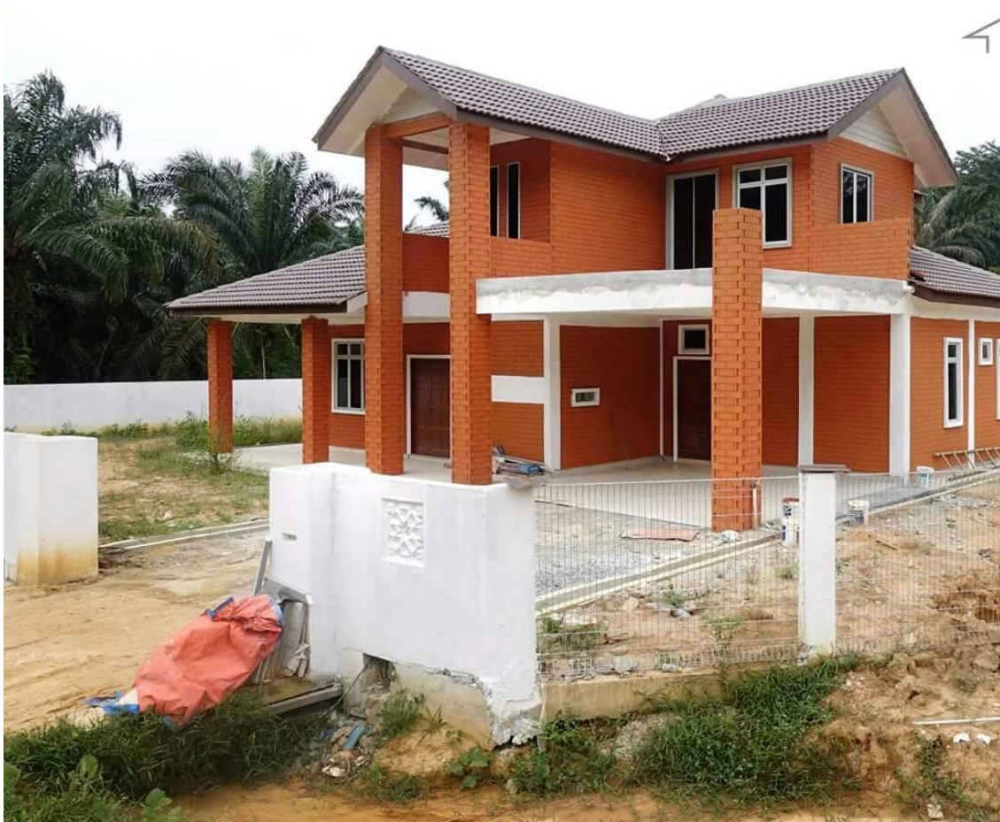
Figure 13: The Two-Floor House at 85% completion. (Source: Millisheid Integrated Services)
