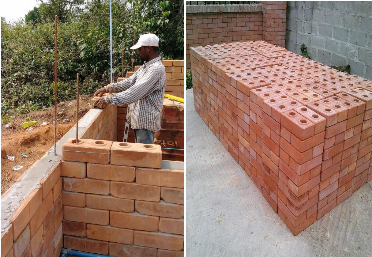
Figure 12: Laying of the stabilized interlocking laterite bricks. (Source: Millisheid Integrated Services)
