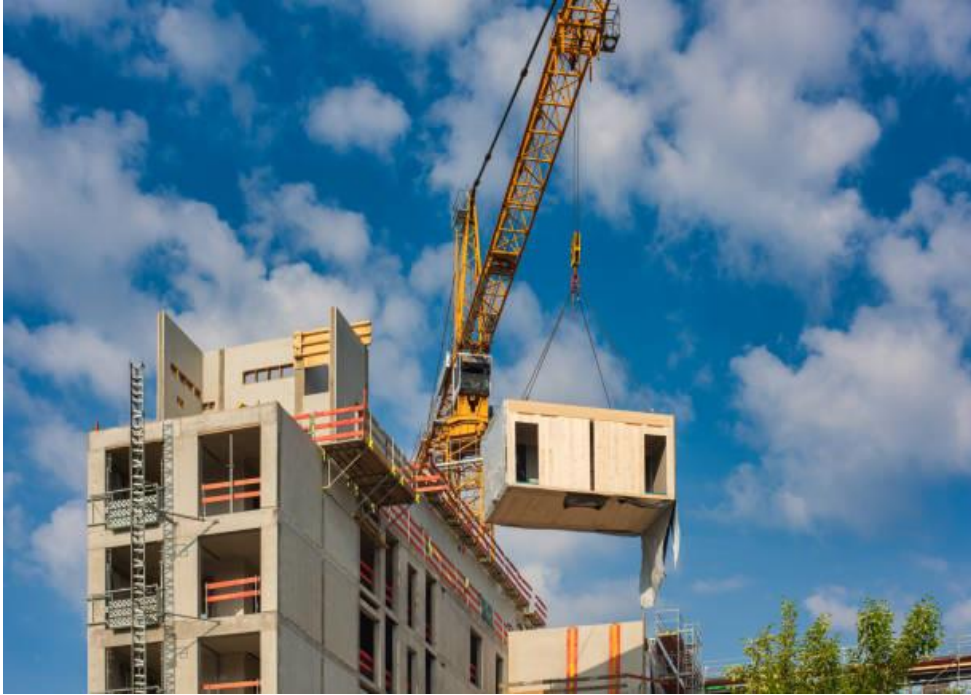
Fig 16: Volumetric modular construction
