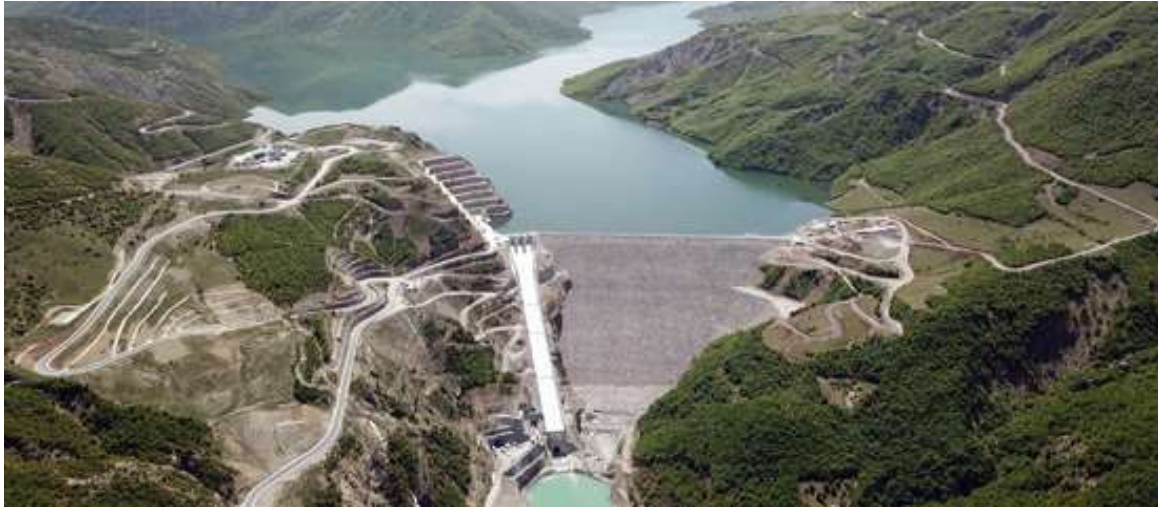
Figure 23: Moglica Hydropower Plant (Statkraft AS, 2020)
