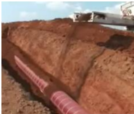
Figure 15. Backfilling of pipeline route /19/
