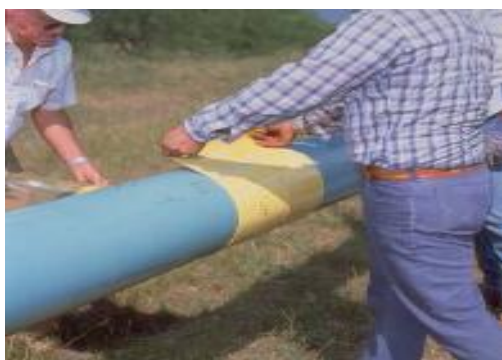
Figure 14. Wrapping a PE tape around a weld joint area /19/.
