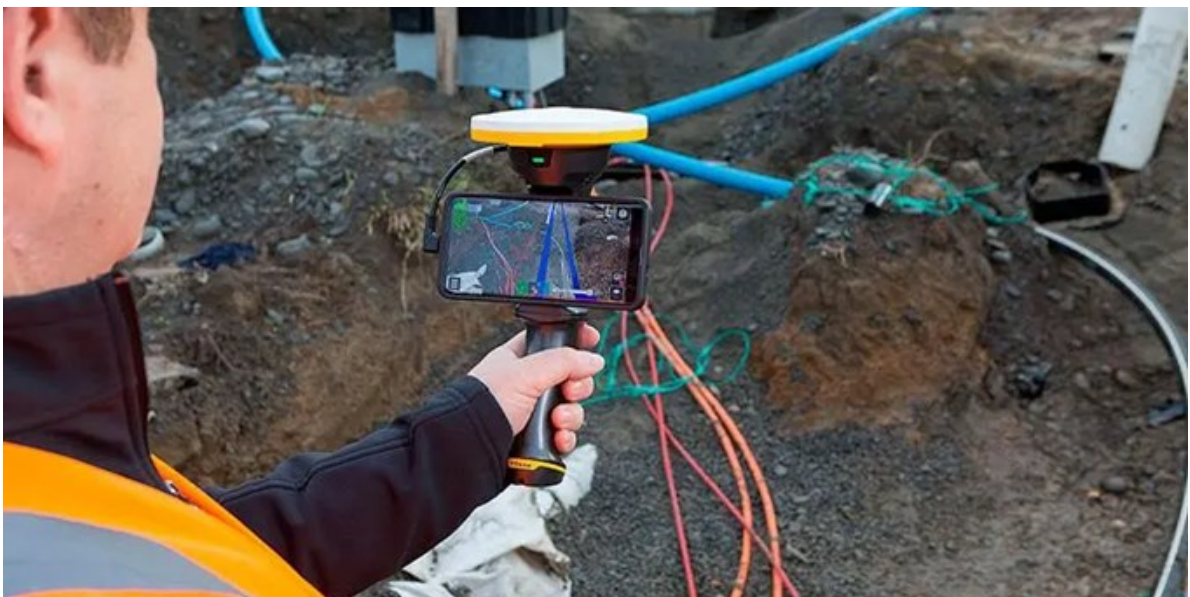
Figur 11. Trimble sitevision (Trimble, 2020).
