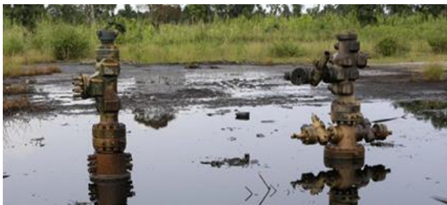
FIGURE 26A. Oil spill in Ogoni land (Friends of the Earth International, 2011)
