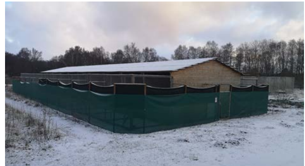
The Stadio Owlímpico research facility at Stensoffa ecological station, Lund University
