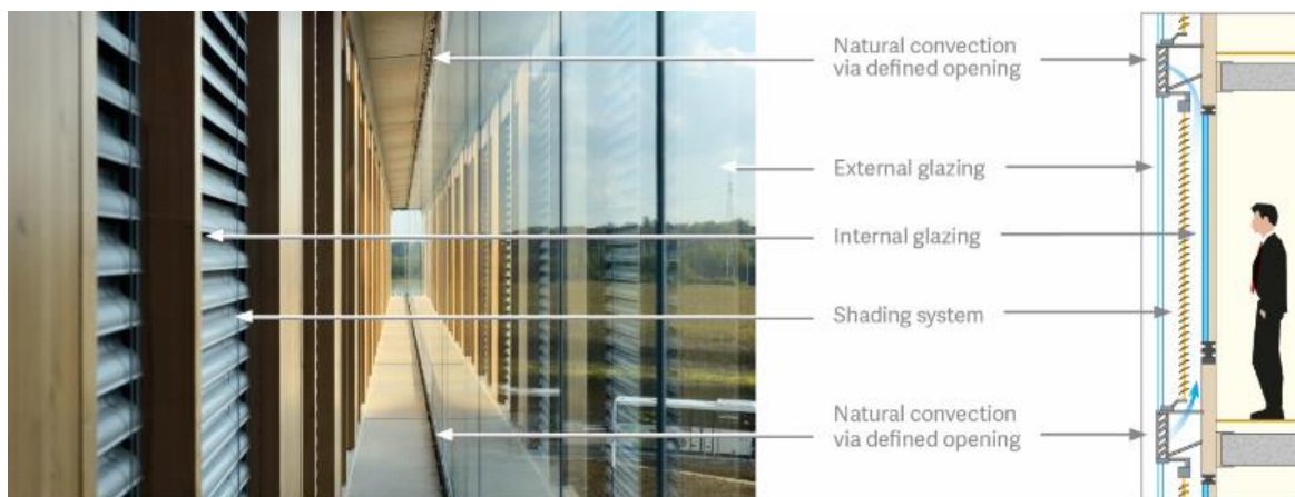
Figur 6. Dubbelglasfasad-koncept (Intelligent Glass Solutions, u.d.).
