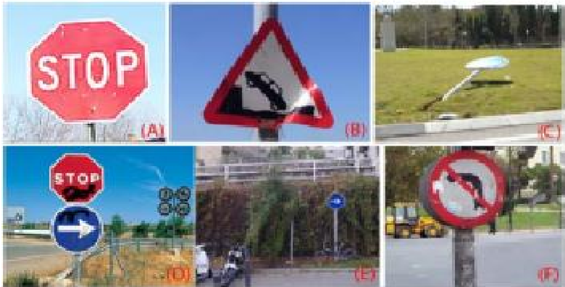
FIGURE 29. Examples of damaged traffic signs (Gonzalez-Jorge, Riveiro, Armesto & Arias)
