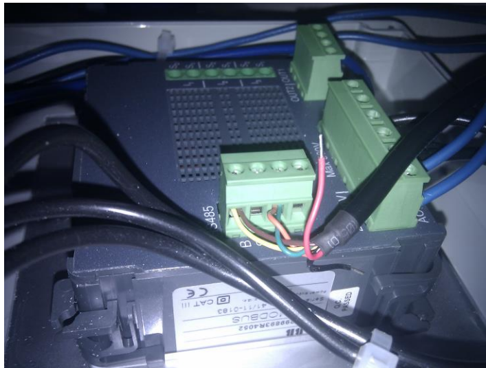
Fig. 28 Wiring of the box and RS485-to-USB converter, A and B pin is used only,
