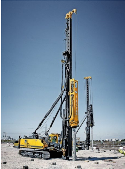
Figure 2. Junttan piling rig.
