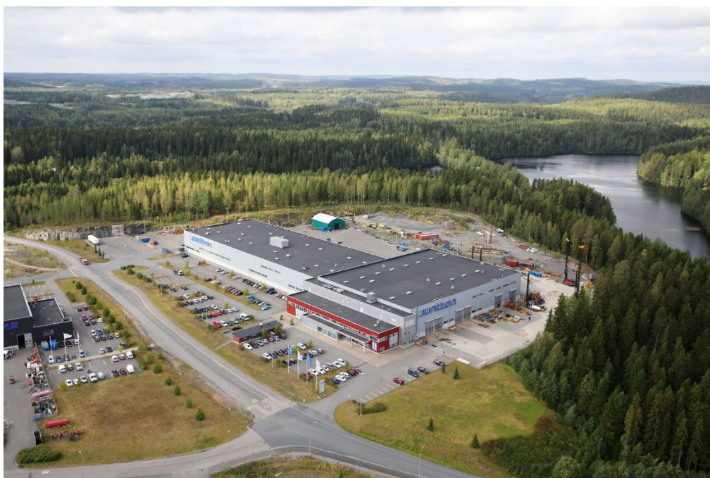
Figure 1. Junttan factory in Kuopio, Finland.
