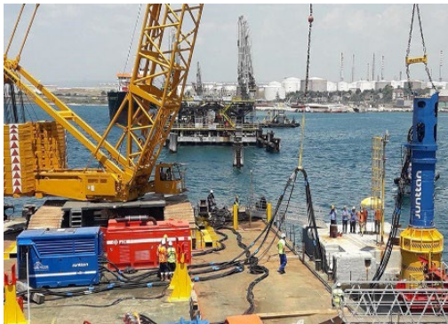
Figure 3. Junttan hydraulic hammer and powerpack.
