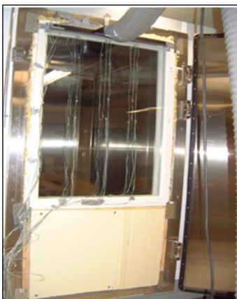
Picture 68. The supply air window in test laboratory in Rovaniemi.
