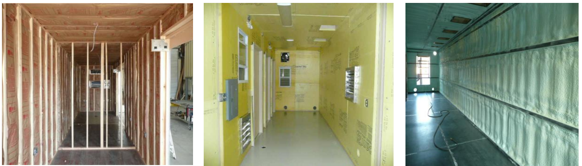
Figure 45: Fiberglass, rigid polystyrene foam panels, and closed cell spray foam respectively (Gregorio, R., 2012).
