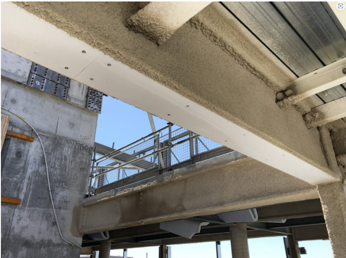
Figure 24. Fire-retardant spray on steel structures. (Progressive materials, 2023)
