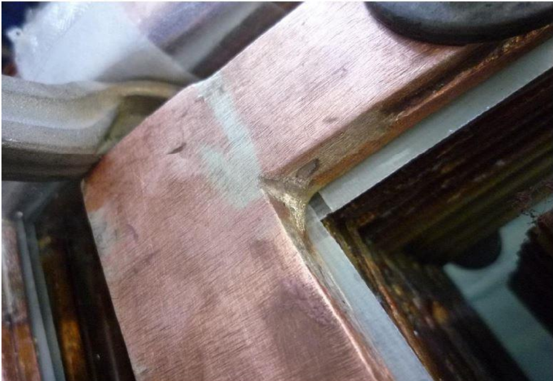
FIGURE 43. New soldered corner connections (19)
