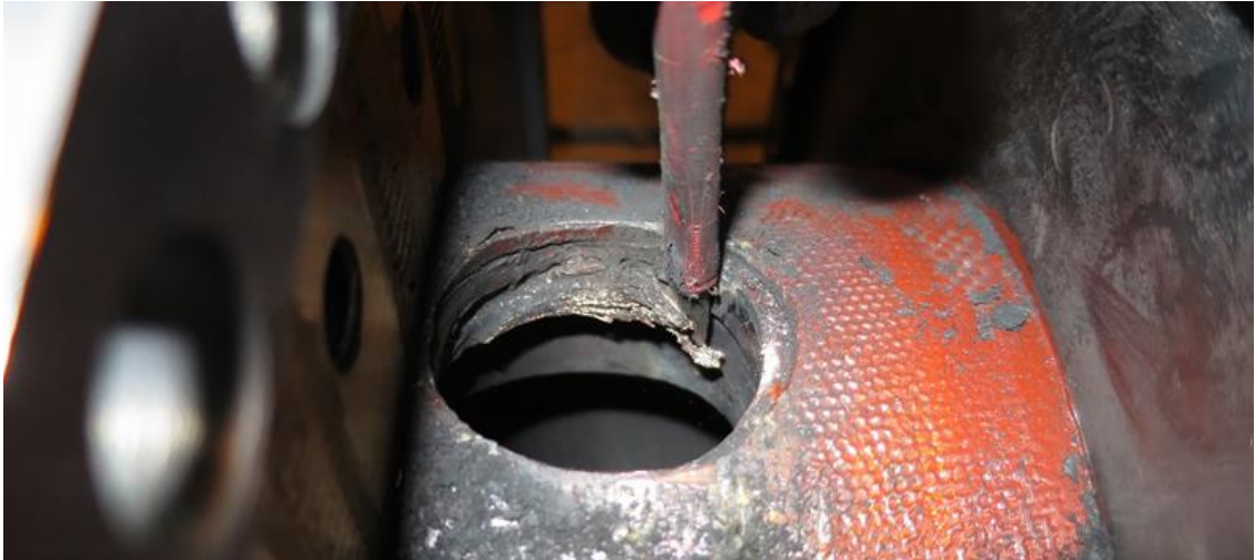
FIGURE 44. Copper in the radial stud hole that caused the ground fault (19)
