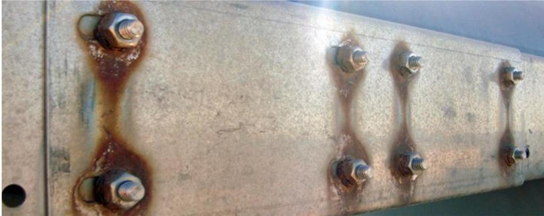
Figure 6: Galvanic Corrosion (Wheeler, 2018)
