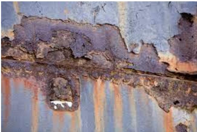
Figure 7: Selective Corrosion (Moriber, 2020)
