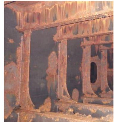
Figure 2: Uniform Corrosion
