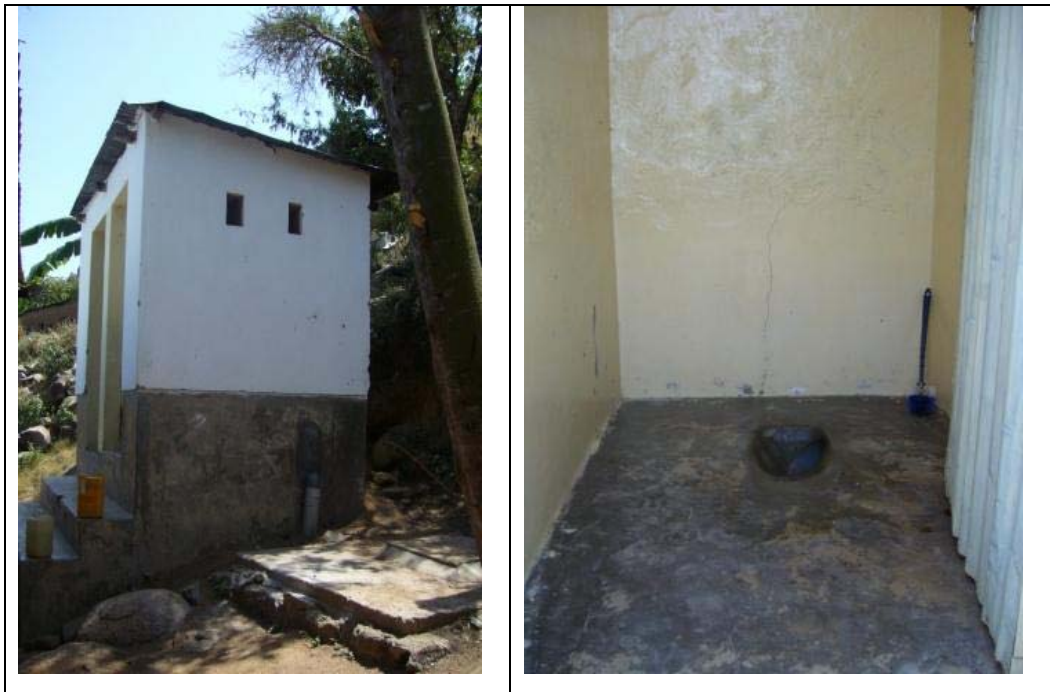
Figure 7. Photos of a mounded pour flush latrine connected to septic tank. The location is at the hills and that is why it is constructed partly on the surface of the ground.
