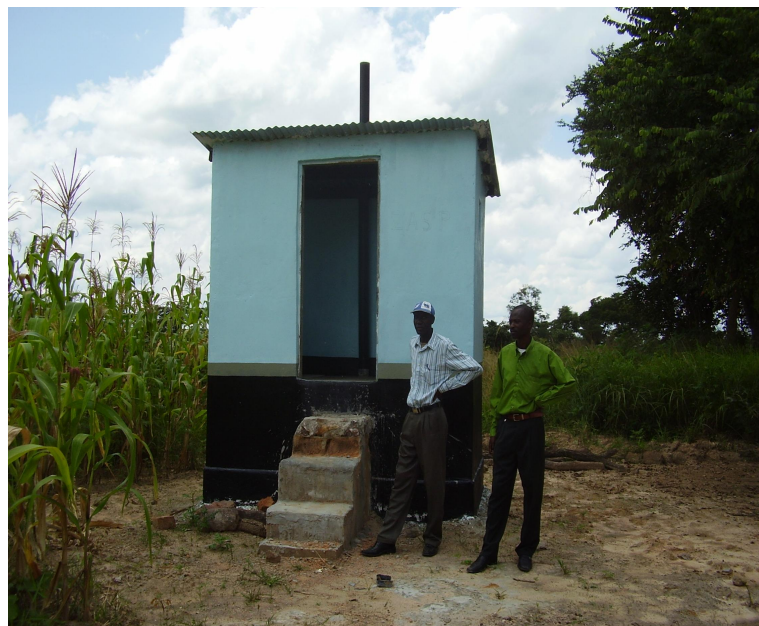
Figure 2. Dry toilet at Kasamwa community
