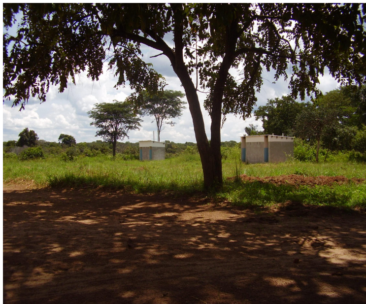
Figure 3. Covered pit latrines at Chisapa community
