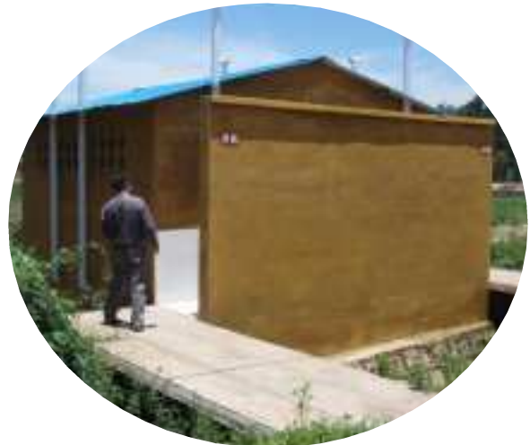
Figure 4: Public urine-diverting dry toilet. Jinning County, 6.08.2007.
