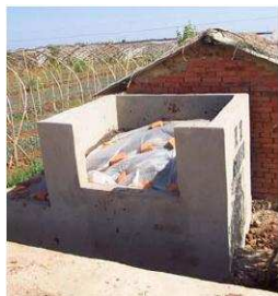
Illustration 3: Dual-chamber composting system. Picture by Wang Hongtao.
