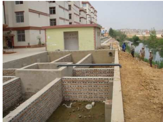
Illustration 5: Wastewater interceptor using biofiltration design under construction. Miikka Ristkari, 2007.
