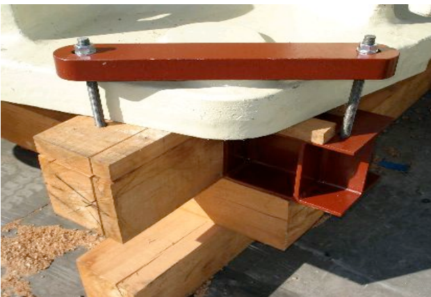
(Pic.93) heavy duty corner bolts to stabilize the main frame.
