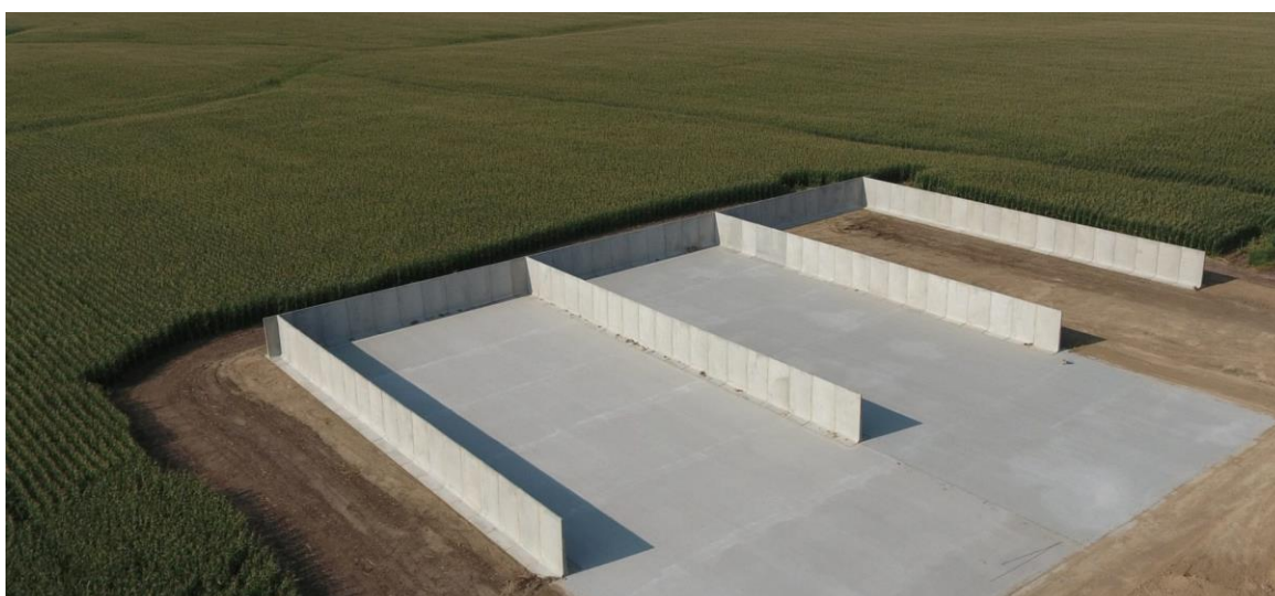
Figure 8. "Bunker Walls". Picture taken from Hanson Silo Company
