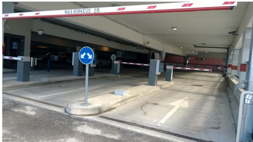
FIGURE 6. Control gates with surveillance device (camera) Paviljonki 1, Jyväskylä
