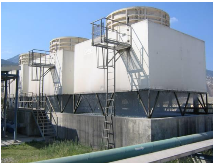
Figure 35. Cooling towers installed on a common concrete basin /15/
