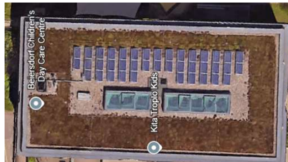
Figure 5.15 Green Roof and Solar Panels (Google Earth)
