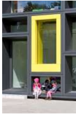
Figure 5.17 Deep Extruded Façade (kadawittfeldarchitektur, 2015)
