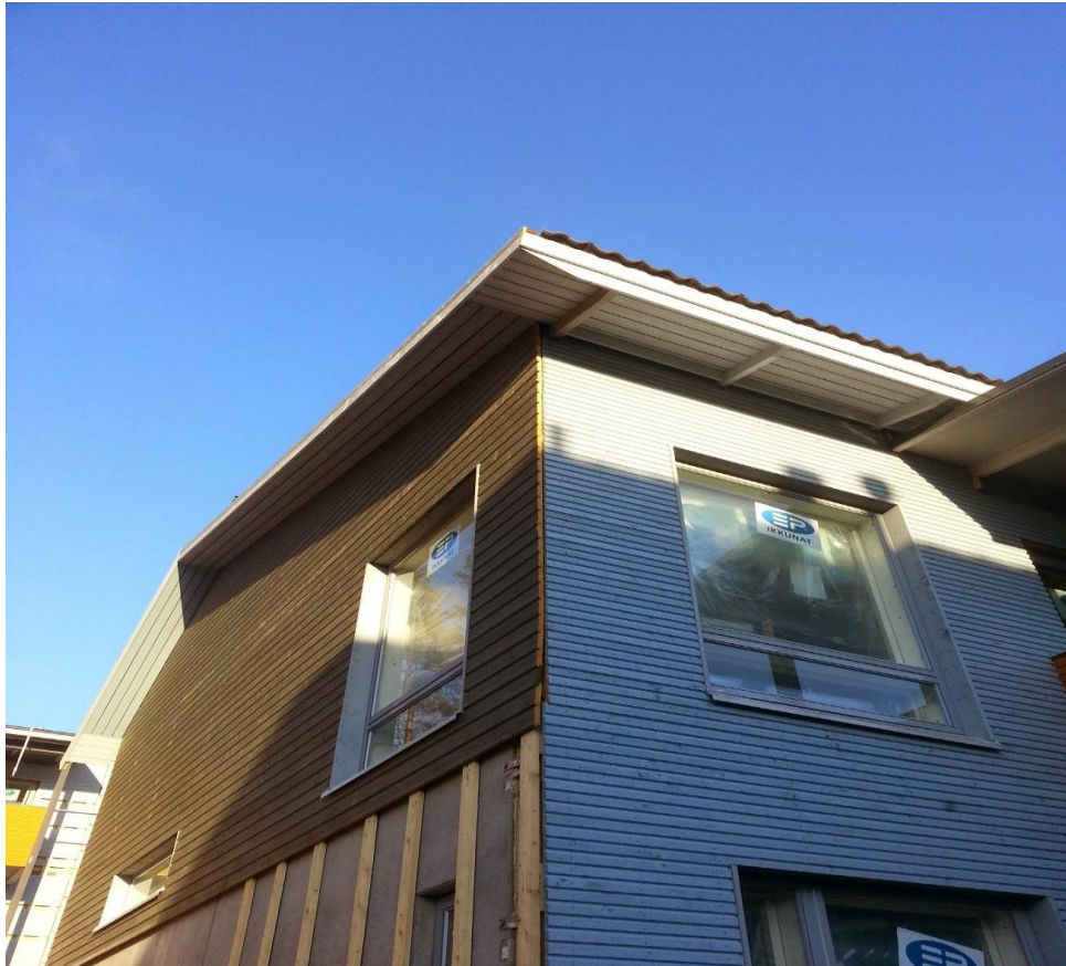
Figure 15 The junction of eaves in building E. Ahokas M. 2014.
