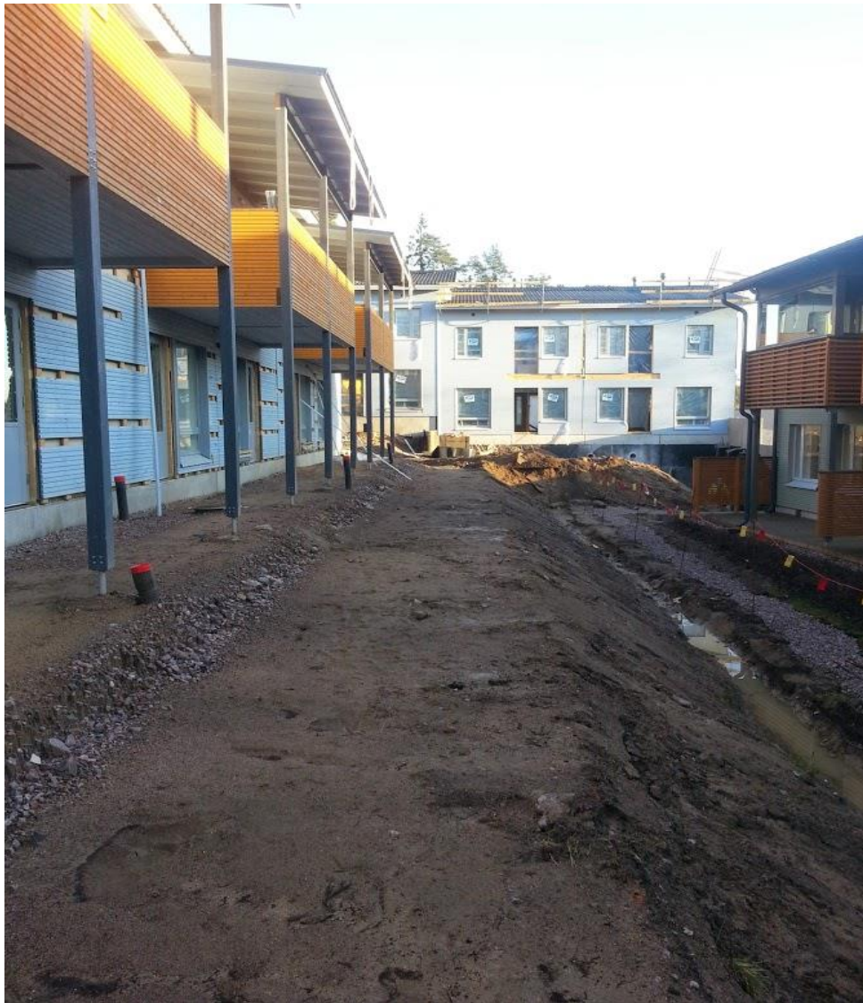
Figure 21 The southern side of building D. Ahokas M. 2014.
