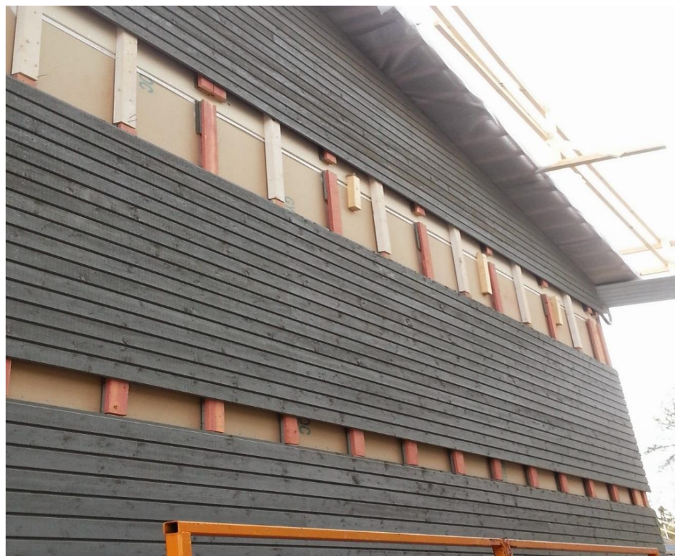
Figure 13 Starting point of the roof woodwork at ends of buildings. Ahokas M. 2014.
