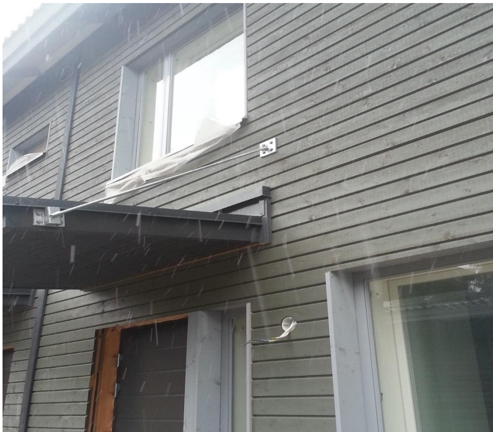
Figure 31 Fixed canopy connection in building F. Ahokas M. 2015.
