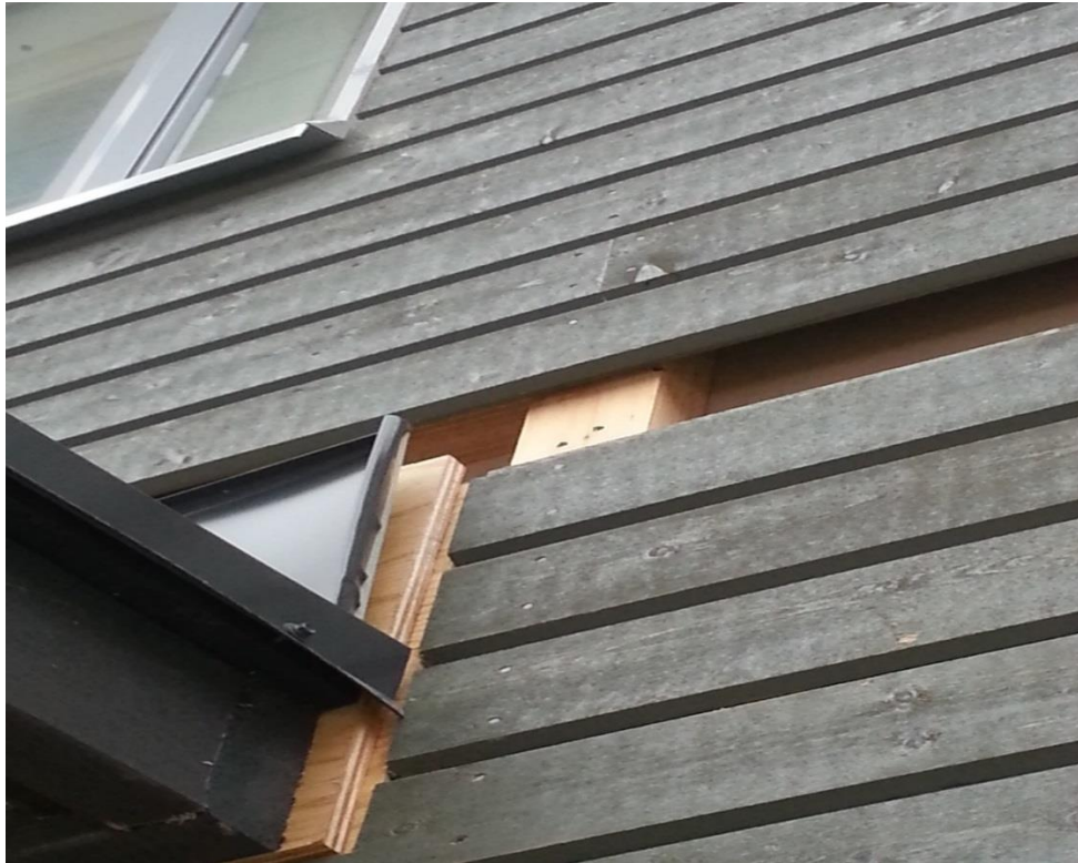
Figure 30 Canopy connection before fixing in building F. Ahokas M. 2014.
