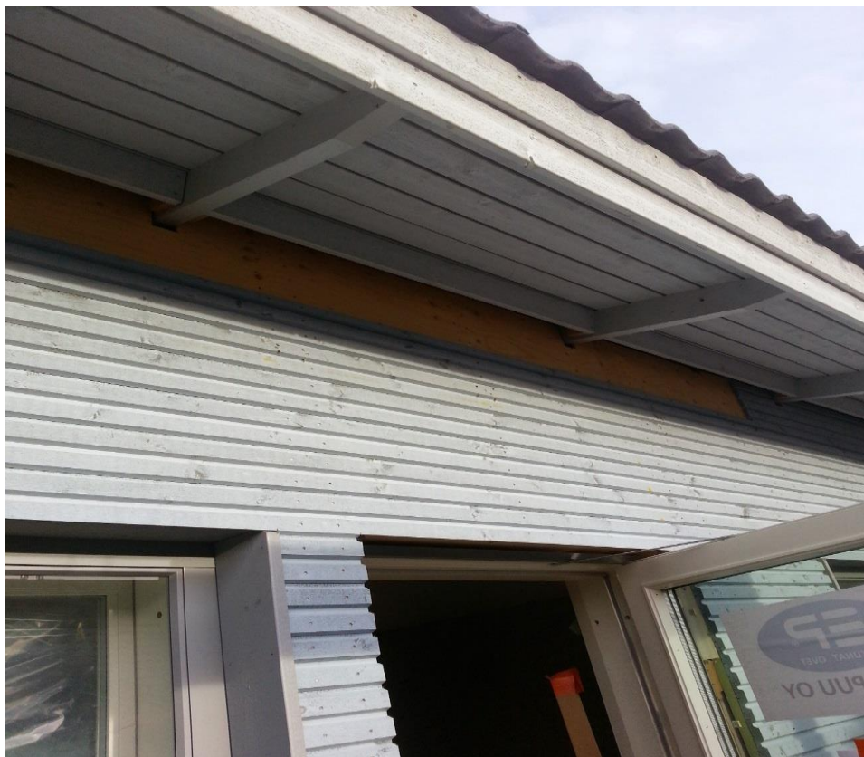
Figure 14 Storm boards and side eaves finished. Ahokas M. 2014.
