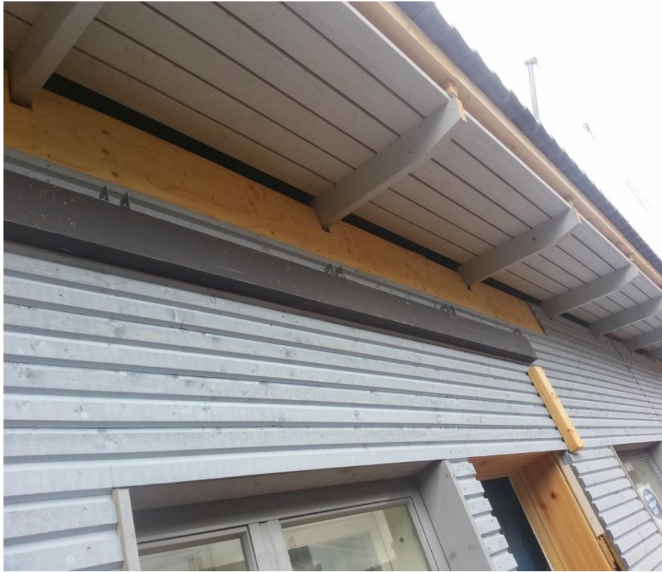
Figure 12 Starting point of the roof woodworks. Ahokas M. 2014.
