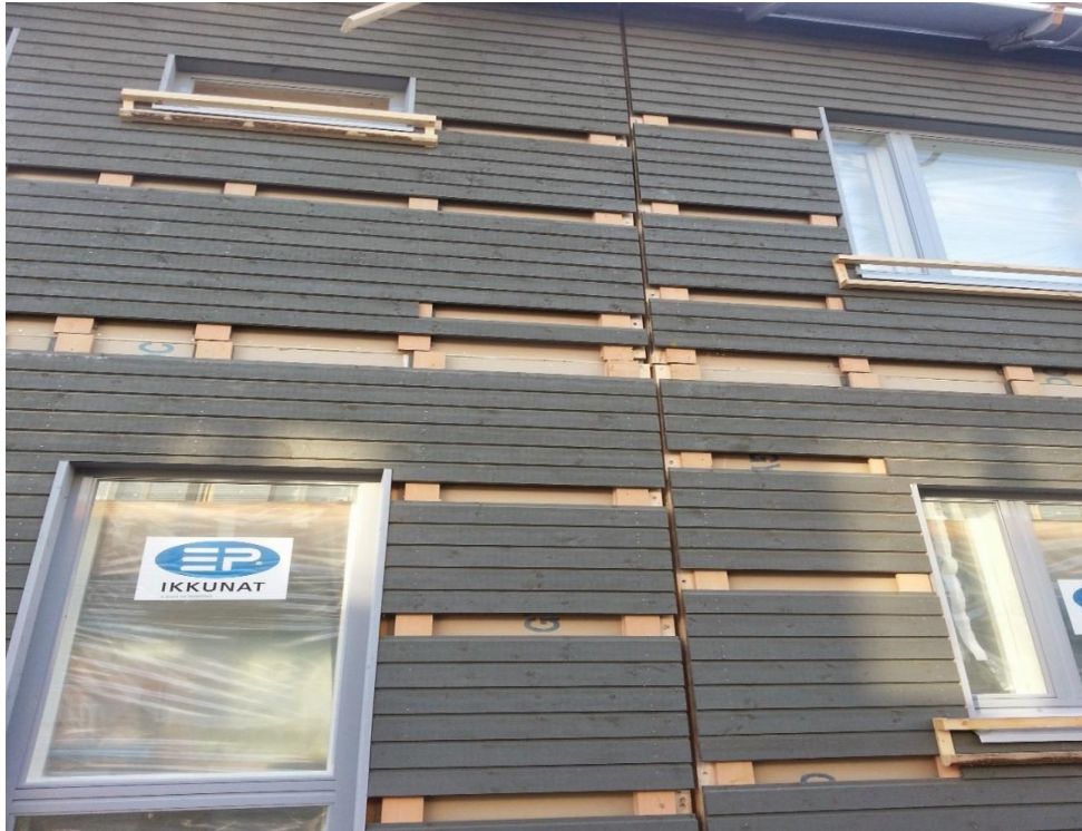
Figure 11 Starting point of façade woodwork. Ahokas M. 2014.
