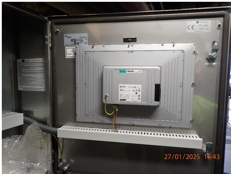
FIGURE 56. Backside of the touchscreen
