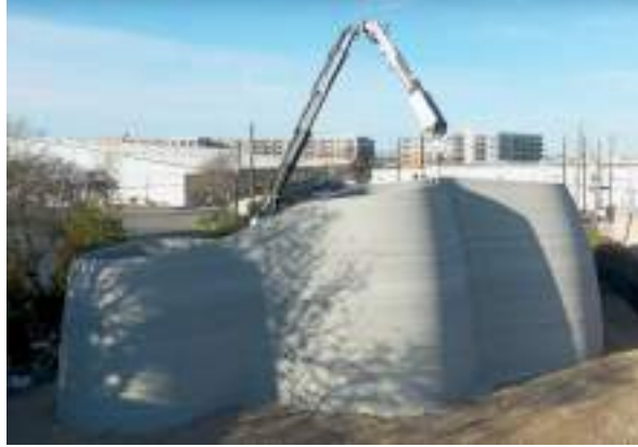
Figure 4: Robotic-arm 3D construction printer (Startup Selfie, 2024)
