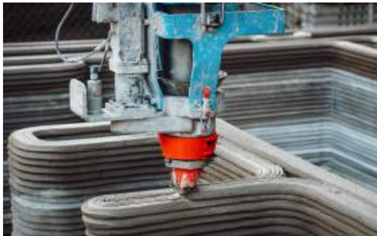
Figure 1: 3D printer extruding cementitious material (Kauppila, 2023)
