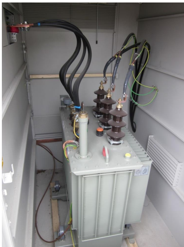
Figur 14 Distributionstransformator i parktransformatorstation
