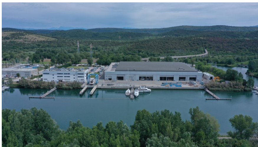
Figure 4 Aerial view of Monfalcone Yard
