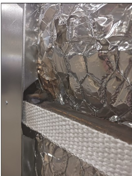
Figure 5. Fiberglass tape attached to the support structure. Photo by author, 2023.
