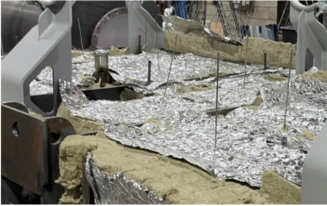
Figure 6. Wool pins sticking up through the wool, at this stage, the points of the pins will be bent down back into the wool. Photo by author, 2023.
