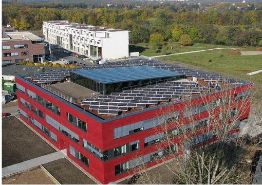
Figure 25. Roof of the Etrium building with PV panels [74].
