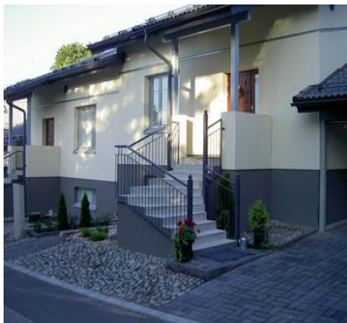
Figure 6. Paroc Passive House, Tikkurila, Finland [34].
