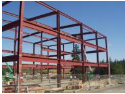
Figure 27 Moment resisting steel frame ( http://www.allstructure.com/projects.htm )
