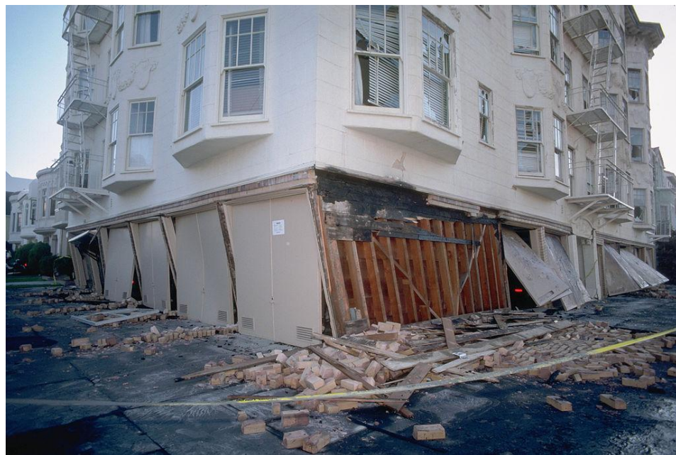
Figure 17 A soft-storey mechanism example ( http://en.wikipedia.org/wiki/Soft_story_building )
