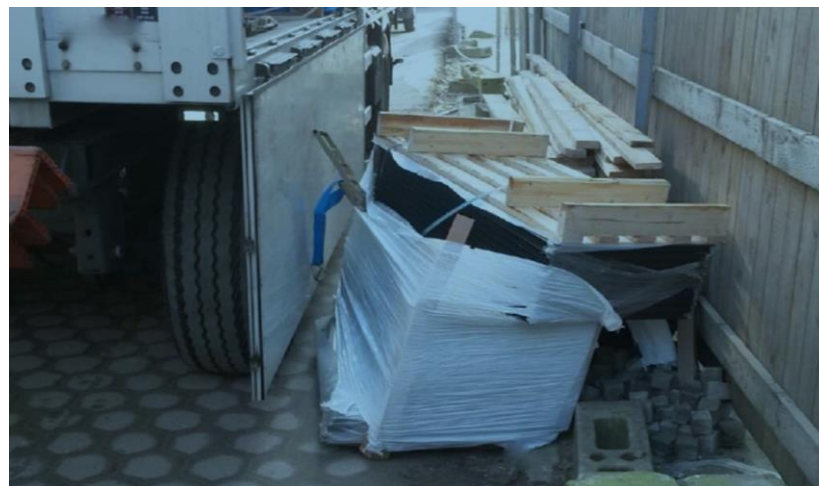
PICTURE 5. Wrong handling – package collapsed from truck due to lack of compliance with instructions
