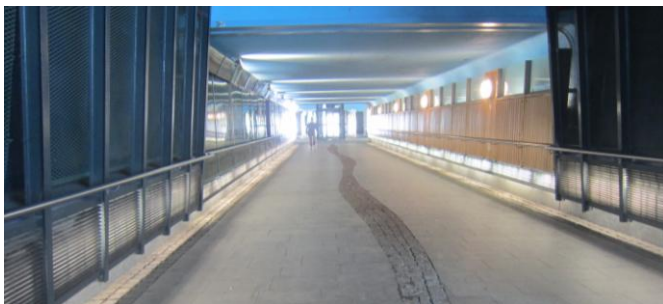
Image 39: The station tunnel under the tracks (Jaakkonen, 2015)
