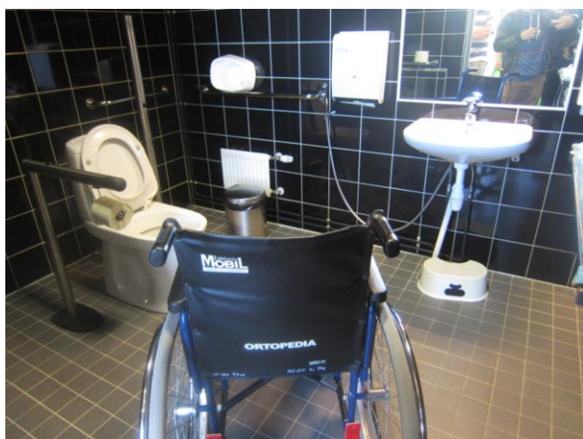
Image 29: The second accessible toilet (Jaakkonen, 2015)
