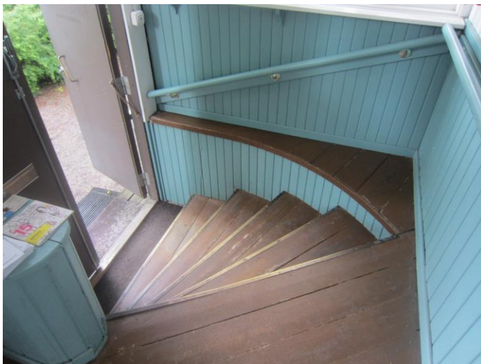
Image 8: Staircase to the Gallery (Toivanen, 2015)
