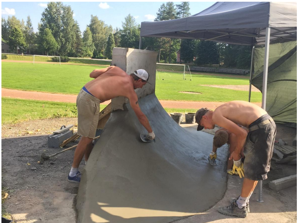
Figure 24 Workers floating a curve by hand. (Windmill Skate Co.)
