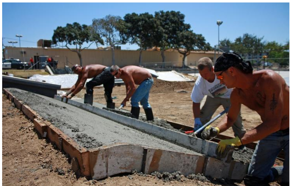
Figure 22 Workers screeding concrete on a bank. ( https://s-media-cache-ak0.pinimg.com/736x/f5/6e/a7/f56ea79252b81eb1f713652a04815d60.jpg )
