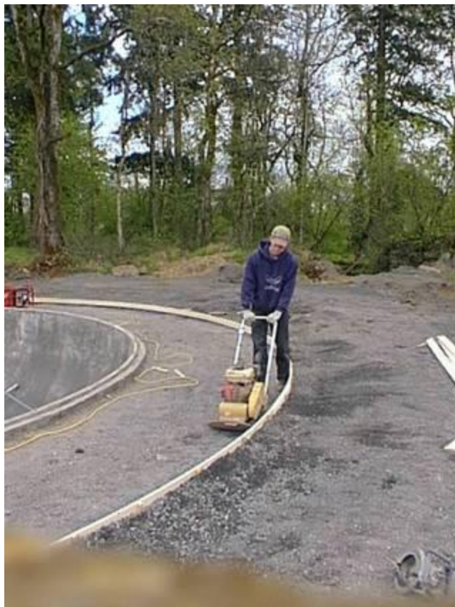
Figure 12 Worker using a compactor. ( http://www.skateparkguide.com/images/articles/19.jpg )
