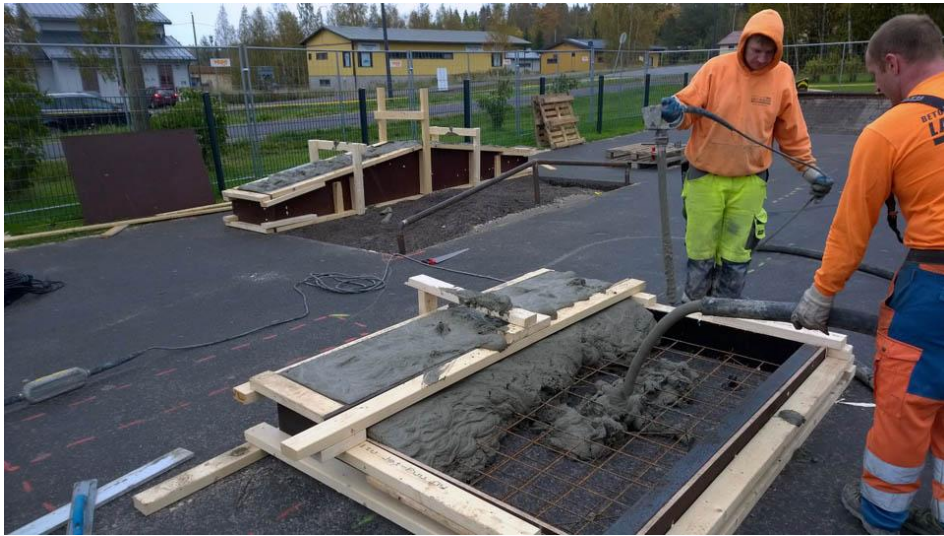
Figure 21 Pouring of concrete at Pornainen skatepark, Finland ( http://www.ebaka.fi/skeittiparkki/sp05.jpg )
