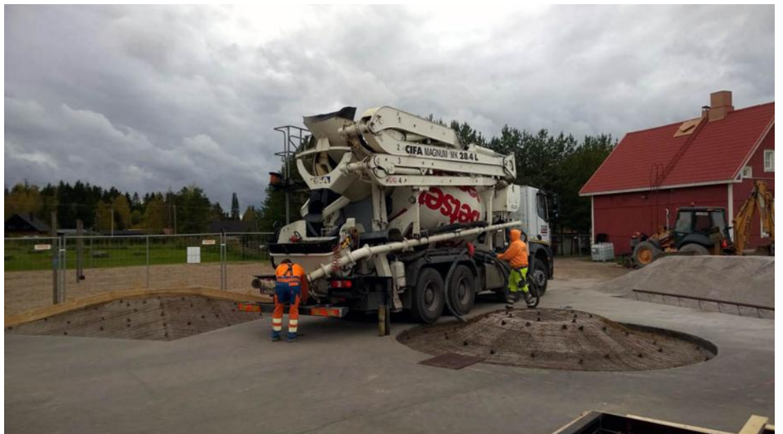
Figure 30 Rebars and connections in place, ready for concreting ( http://www.ebaka.fi/ )
