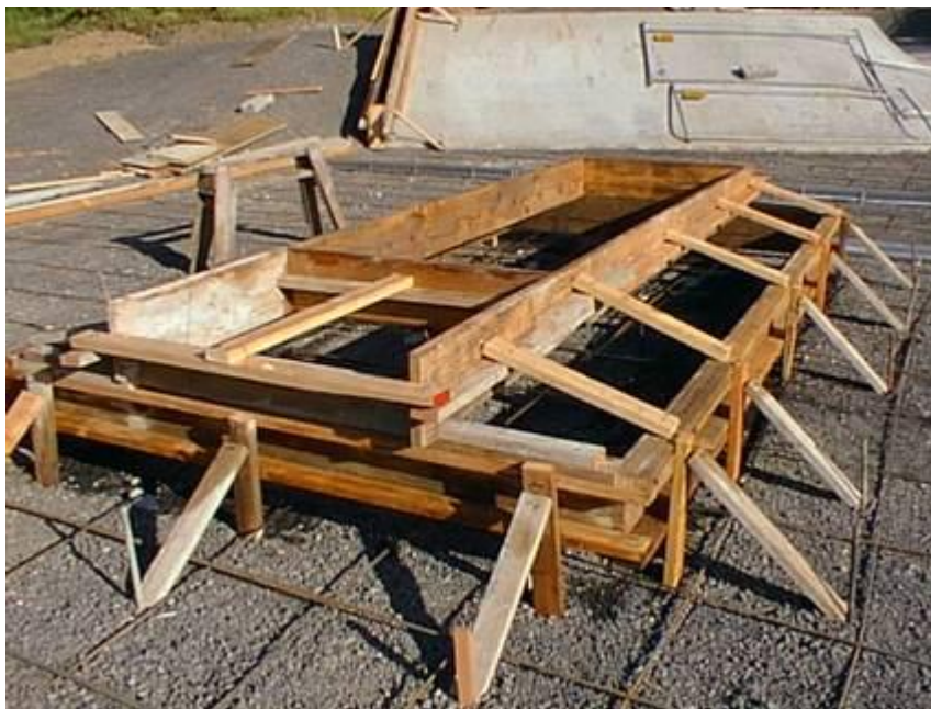
Figure 20 Formwork of a funbox ( http://www.skateparkguide.com/images/articles/5.jpg )
