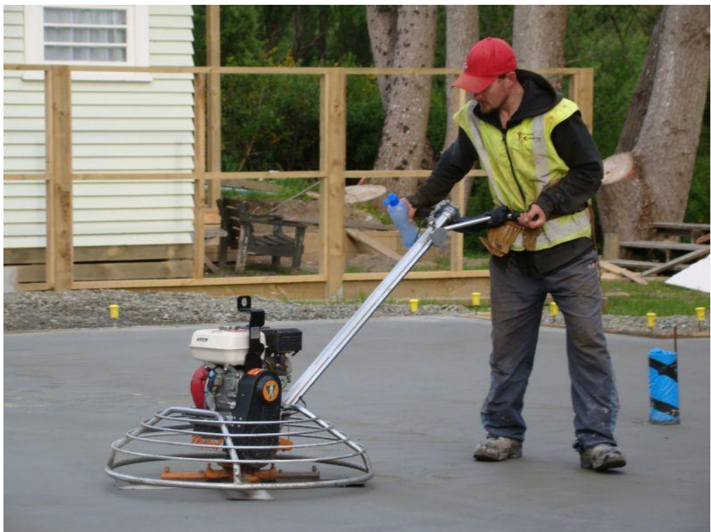
Figure 27 Worker using a power trowel. http://www.bluestone1.co.nz/files/cache/cec866d03b71f5a94d8439c185419df3.JPG
