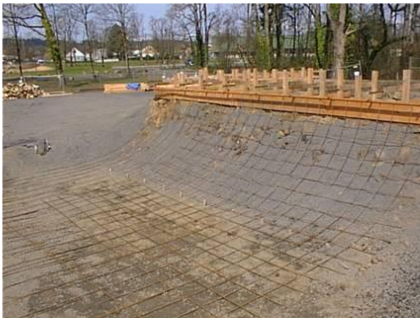
Figure 17 Reinforcement of a quarter pipe. ( http://www.skateparkguide.com/images/articles/32.jpg )
