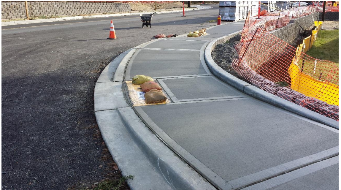
Figure 19 Expansion joints in a sidewalk ( http://www.customconcrete.biz/Portals/119041/images/ )
