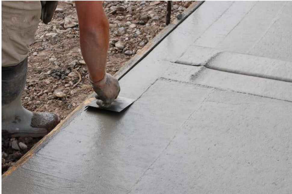
Figure 25 Worker using an edging tool. ( https://www.icreatables.com/images/exteriorhomeimgs/concrete/concrete-edger.jpg )
