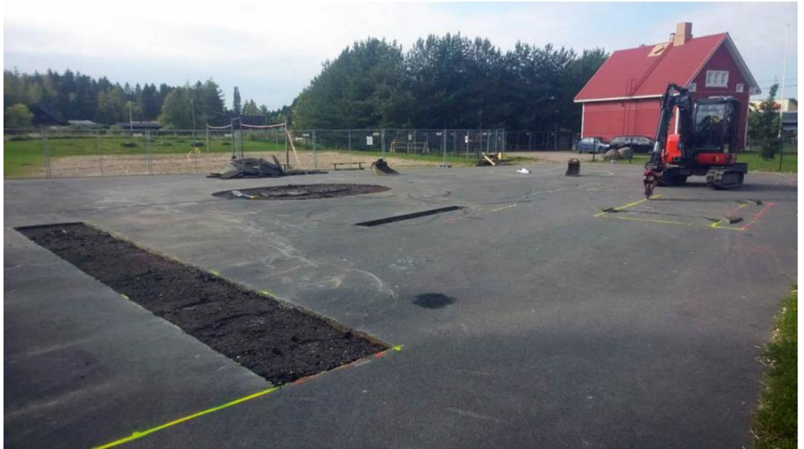
Figure 29 Excavator cutting slots in the asphalt for concrete obstacles ( http://www.ebaka.fi/ )
